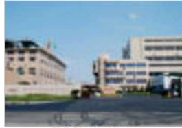
TBR Plant in Xiasha
